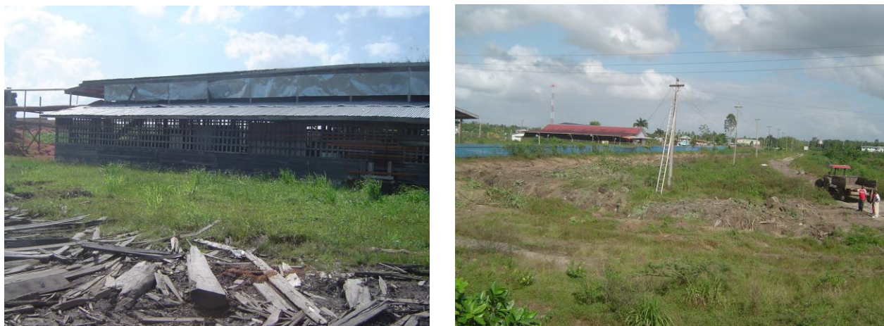
Figure 7: Secondary processing shed and the fence that would have to be relocated.
