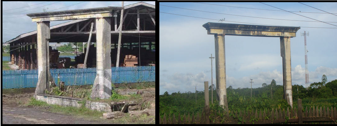
Figure 2.4 River Sluice to be reactivated
