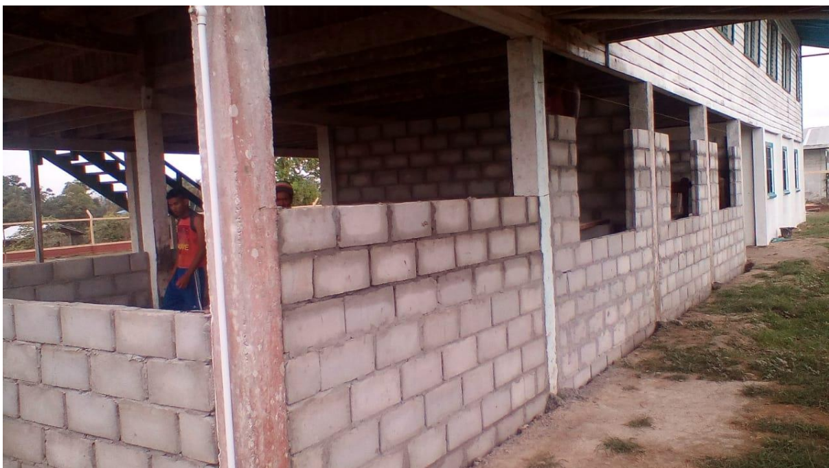
Construction of ICT Hub Facility, Kimbia (Region 10)
