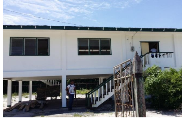
Figure 96 - Multipurpose Center (Region 2)
