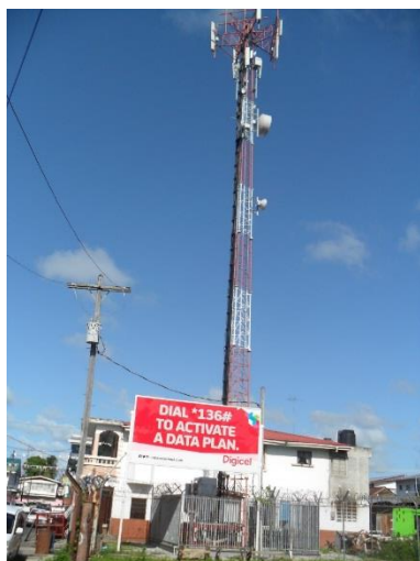
Figure 167 - Digicel Antenna (Region 4)
