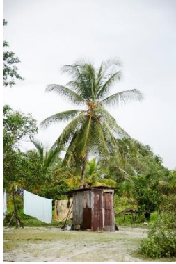
Figure 63 - Pit latrine with slab (Region 4)
