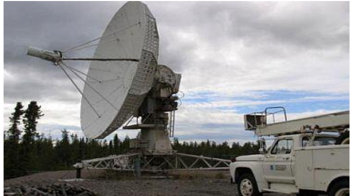
Figure 267 - Satellite ground station for professional operators, also used as Sat-backhaul per site
