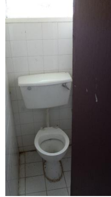
Figure 64 - Toilet linked to sewer (Region 3)
