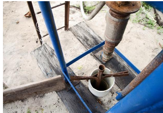
Figure 60 - Drilling for water (Region 4)
