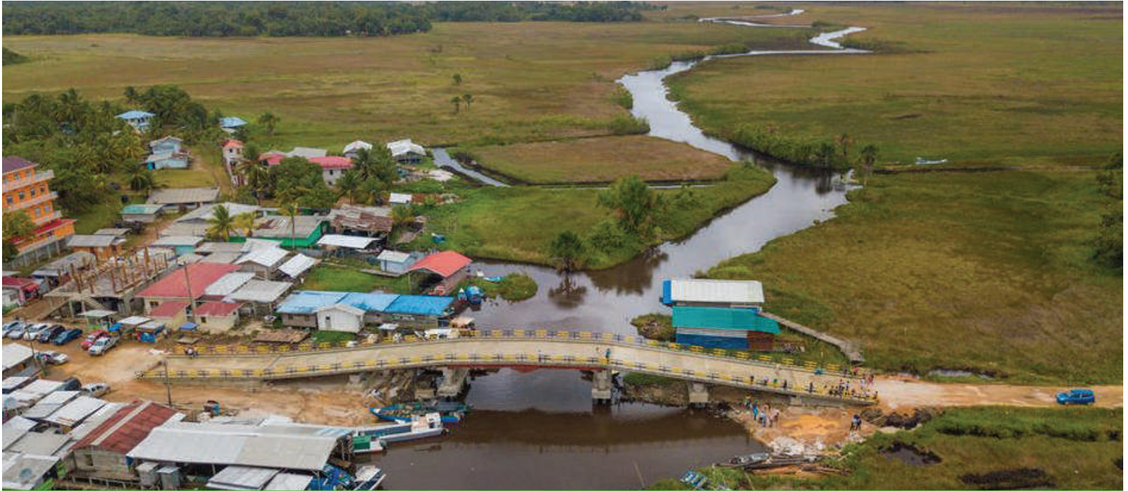
Moruca Bridge. Photo Credit: Department of Public Information
