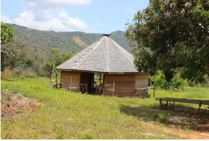
6 Under Construction Karasabai Nature Tourism Project
