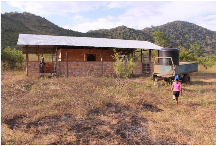
7 Tiger Pond Cassava Processing Building under Construction
